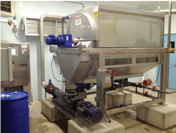
Rotary Drum Thickener
